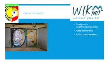
GPON is ideal for multi-apartment housing, but also for individual users, As you can see on picture: We install the fiber optic distribution box in the building, and subscriber cables, also main part of GPON already mentioned optical splitter.
